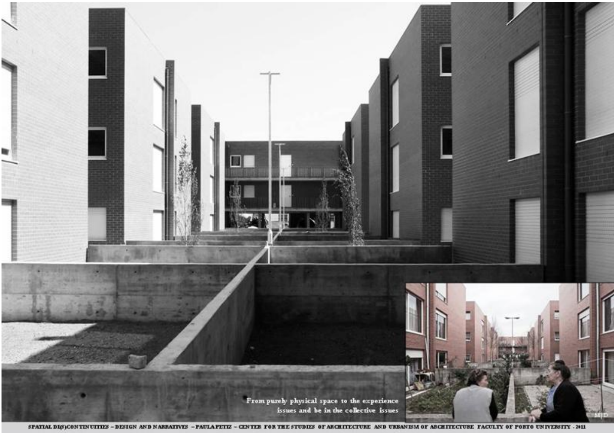
SPATIAL DISCONTINUITIES - DESIGN AND NARRATIVES - PAULA FETIZ - CENTER FOR THE STUDIES OF ARCHITECTURE AND URBANISM OF ARCHITECTURE FACULTY OF PORTO UNIVERSITY - 211
