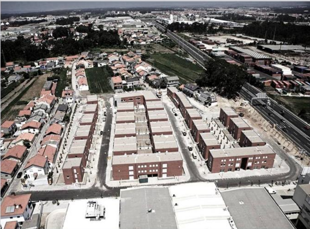
SPATIAL DISCONTINUITIES - DESIGN AND NARRATIVES - PAULA FETIZ - CENTER FOR THE STUDIES OF ARCHITECTURE AND URBANISM OF ARCHITECTURE FACULTY OF PORTO UNIVERSITY - 2011
